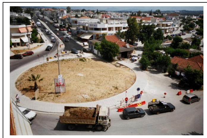
Fig. 1. On the upper right point of this roundabout, a small house resists demolition of the Porta Messinià . Cars are entering the moat road.
